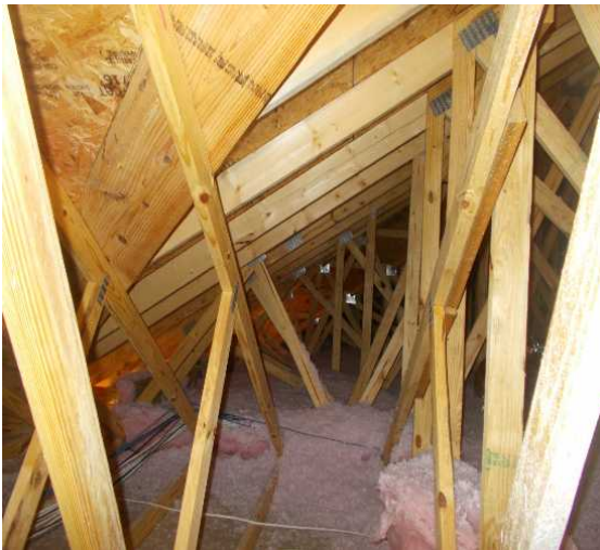
Trusses in the attic.
