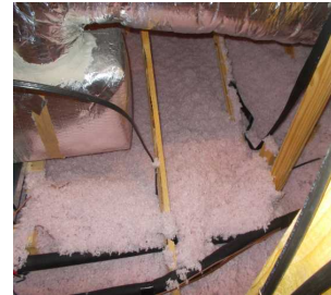
Insulation in attic.
