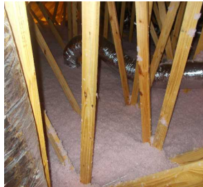
Insulation in attic.
