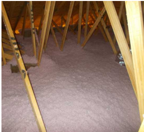
Insulation in attic.
